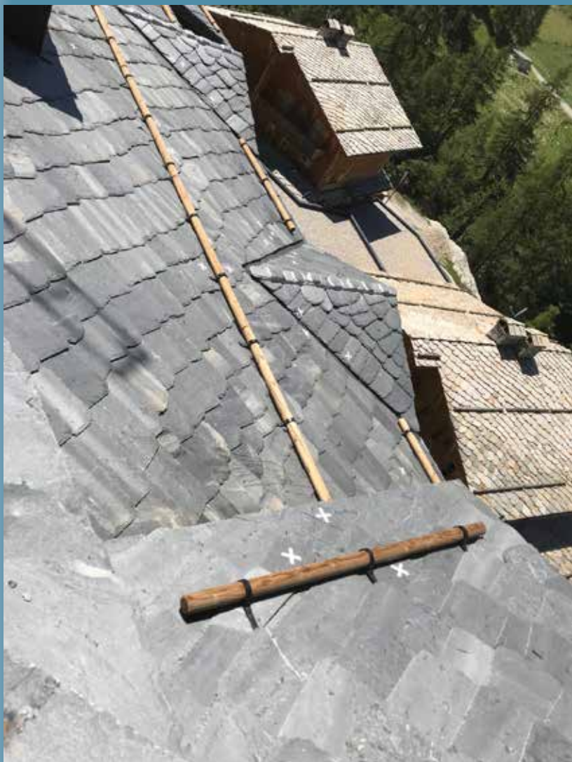
Losette alla valdostana in Quarzite Norvegese - Lauzes opus-incertum en Quartzite de Norvége Polygonalplatten für Dach Alta Quarzit - Norwegian quartzite irregular roofing slabs
